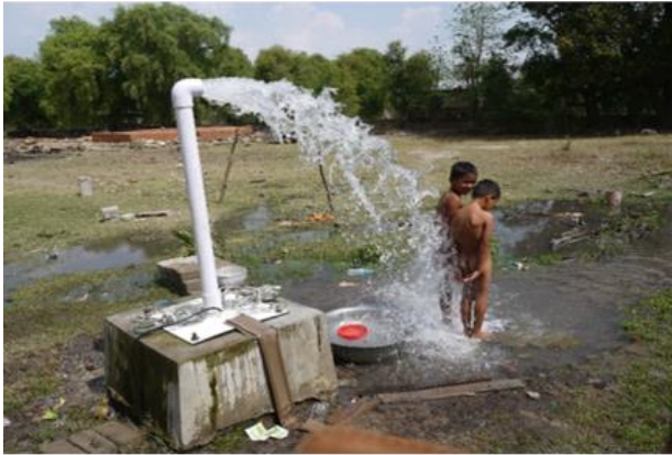
The moment of initial installation
