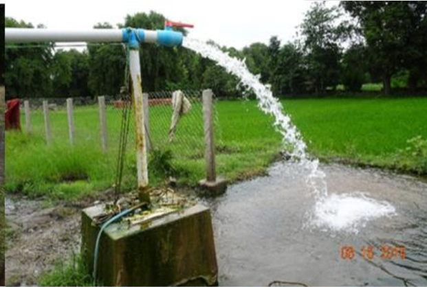
3-month after the installation
